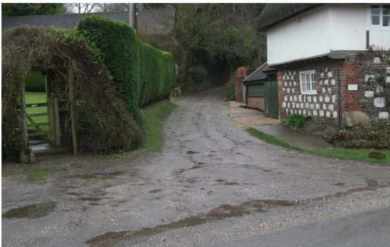
View of western end of Durnford 4 (Woodrow) past Woodrow Cottage
